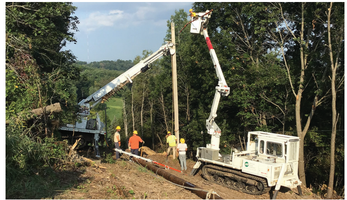
Another project for 2022 was building a tie line between Frenchville and New Amsterdam substations. This is part of a three-mile long re-build project along Hwy. 54/Silver Creek Road and ending at the intersection of Gillmeister Rd./Crystal Valley in the Galesville area. The right-of-way clearing was done by our contractor, Zielie's Tree Service.
